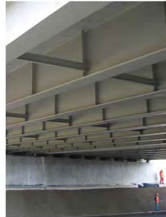
Highway bridge - Lovosice
