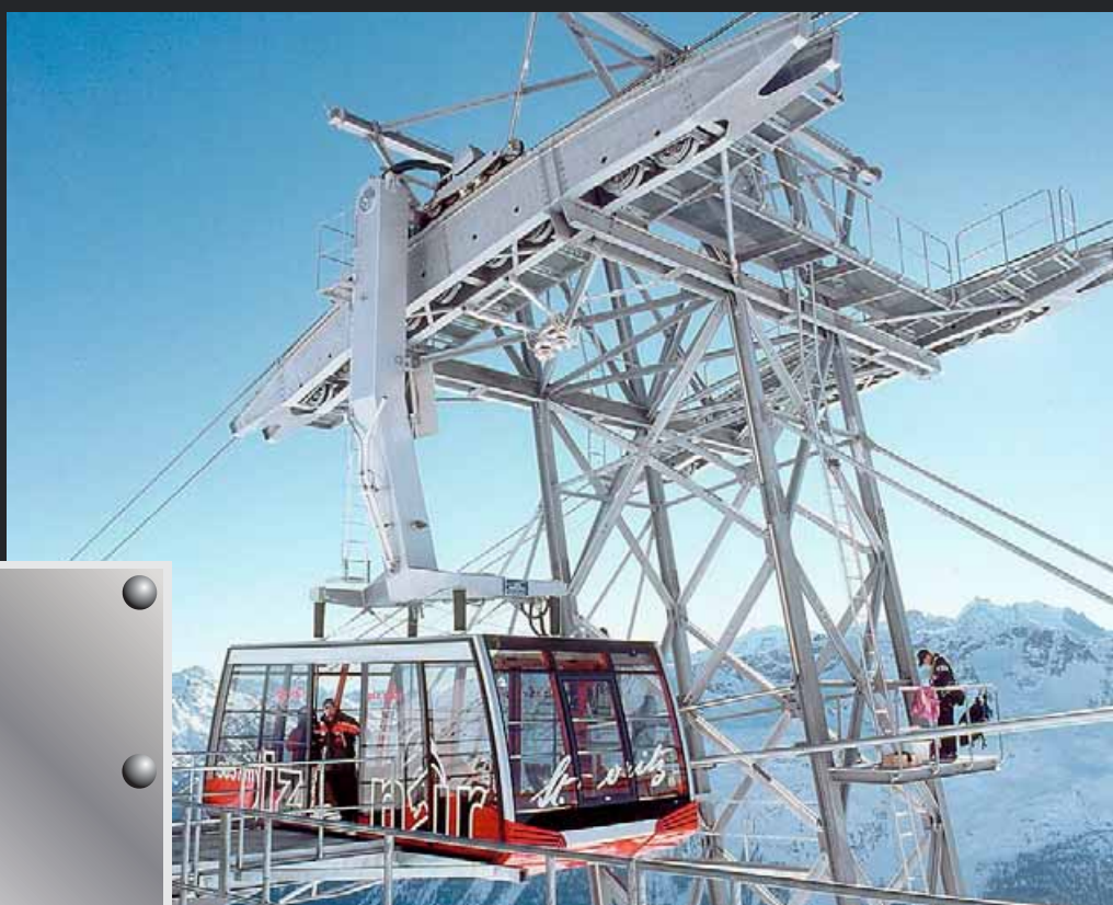
Lattice cableway mast manufactured by EGE spol. s r.o.
