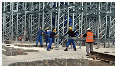
Construction of freezing warehouses for Galliker in Switzerland.
