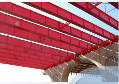
In 2013 a new section of the R7 highway will open running from Droužkovice to Nové Spořice. The overpass is designed as a steel-concrete composite structure consisting of steel welded beams coupled with reinforced concrete slabs.
