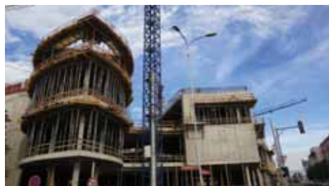
Reinforcing steel supply to the company FERI, s.r.o. Hradec Králové.
