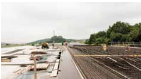
Reinforcing steel supply to the company STAV-TECH-CAR
